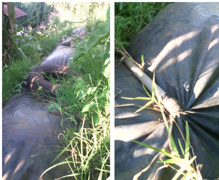
Plastic Tube Biodigester System
