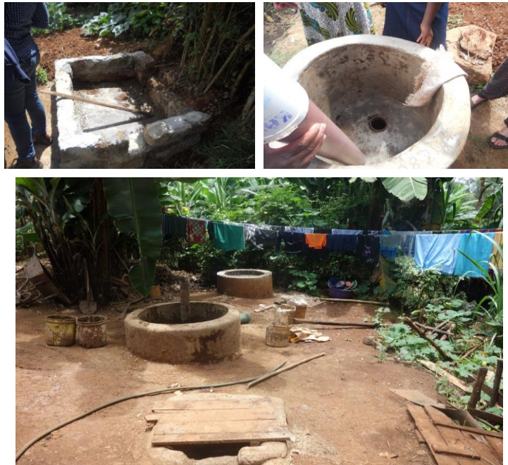
Fixed Dome Biodigester System
