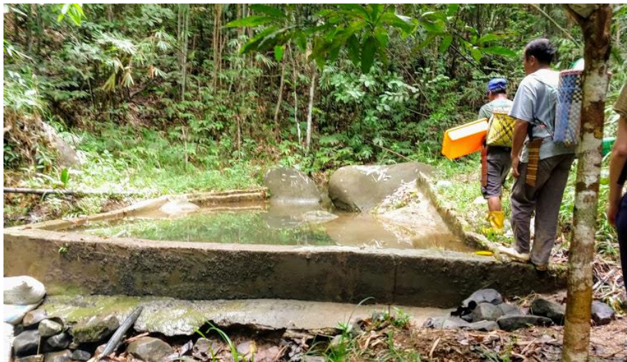
The gravity feed water system reservoir, leading water to the longhouse
